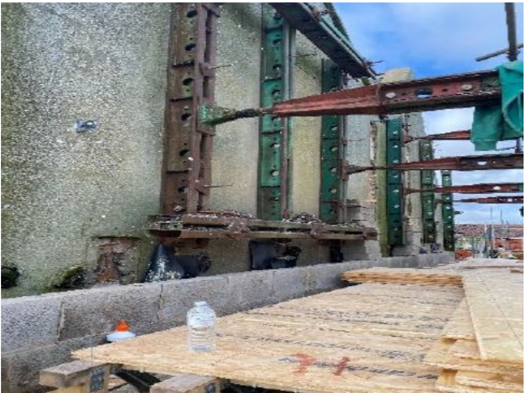
Third floor blockwork progressing
